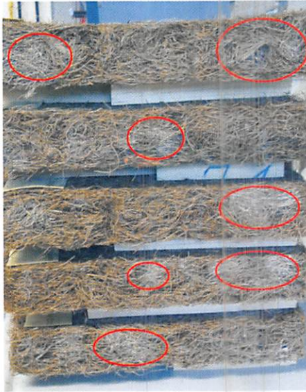
Figure 5. Presence of carbonation spots (red circles) on insulation material made from EFB fibres
