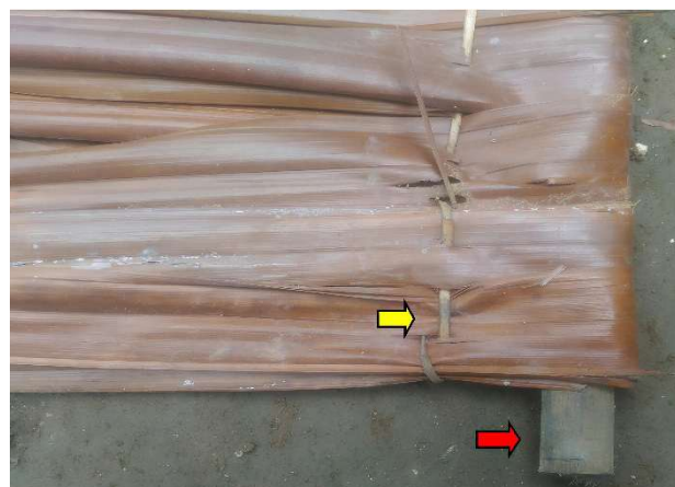
Figure 6. Ato with the main support pole from bamboo culm (red arrow) and rope from sliced rattan (yellow arrow)
